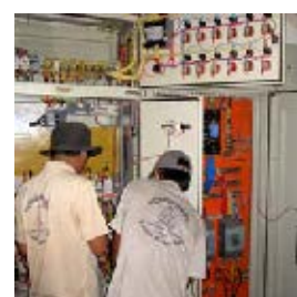
Installing and testing the electrical cabinet for the enterprise
