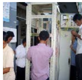
Setting up of electrical cabinet
