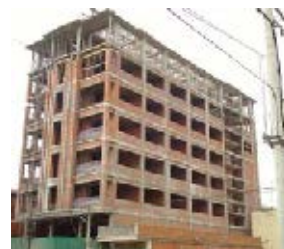
Equipment of this hotel in Battambang
